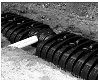
All-in-One as mid-line connection.
