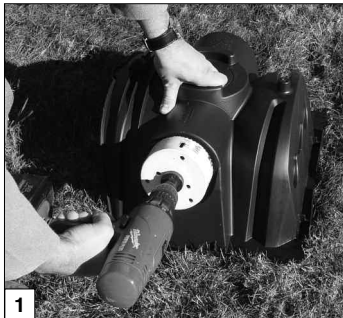
Drill endcap on side or top.
