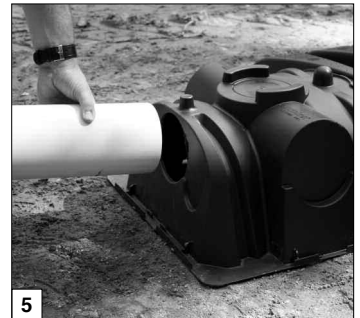
Insert inlet pipe.
