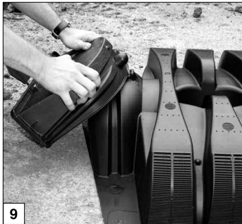
Place end cap outlet end.
